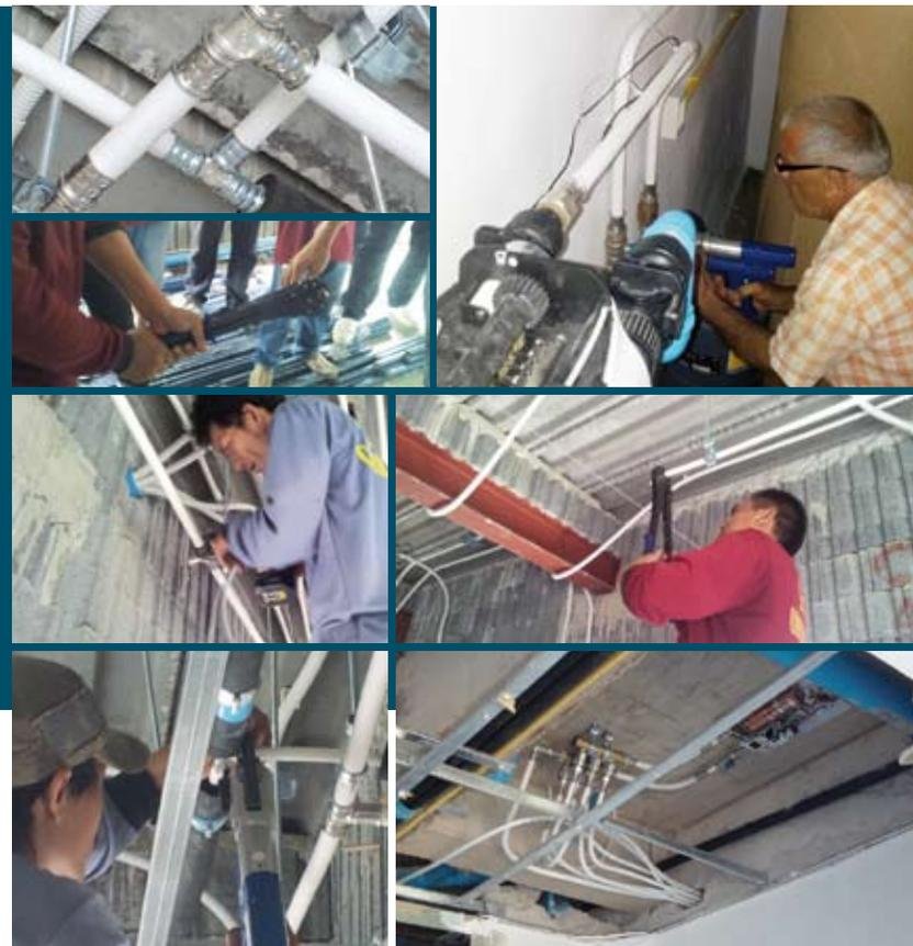
Changing the leaking installation of a nearly ready house by "surgical interventions". The flexible multilayer pipe of MULTITUBO systems minimized the damage for the owner considerably.
